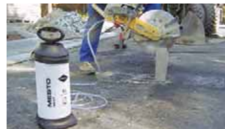
Cut-off grinder in road construction
